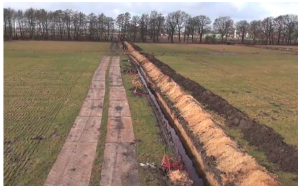
Permanent field monitoring: trenches for permanent receiver lines and one month after installation, Schoonebeek, the Netherlands
